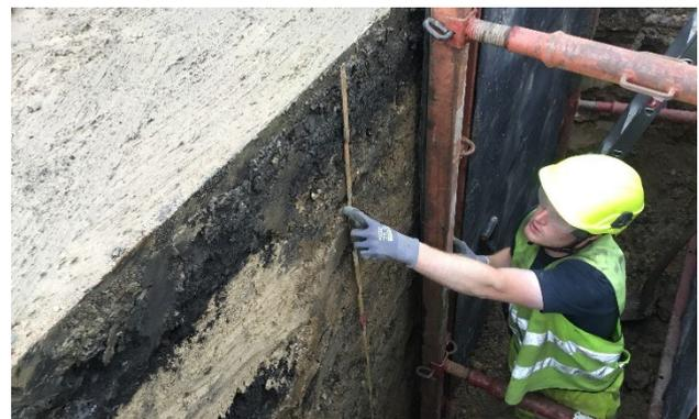
**Fig. 13: At certain places it might be necessary to install the cables very deep, in order to ensure clearance distances to other infrastructure.**
