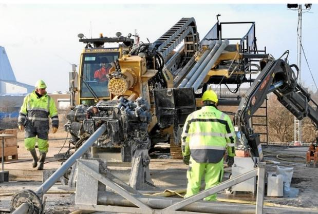
**Fig. 10: The big HDD machine was needed for performing the more than 950 meters HDD drilling.**
