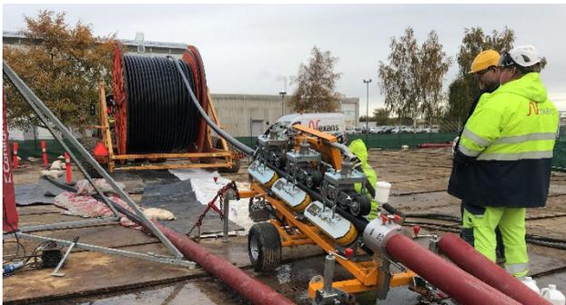
**Fig. 15: Installation of cables using water pressure and caterpillar.**
